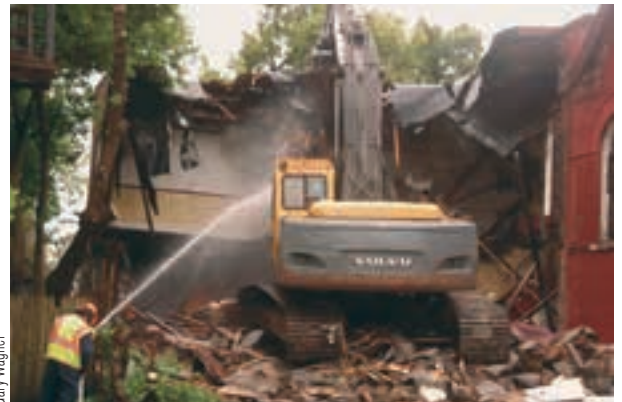
City equipment demolishes a portion of Utica, New York's Karen Adventist Church building to access collapsed sewer pipes for repair.
